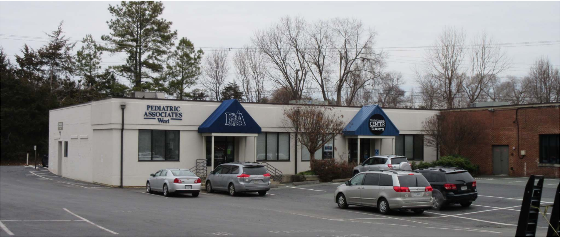
2405 2409 IVY RD – STUCCO FAÇADE & PAINTED CMU
