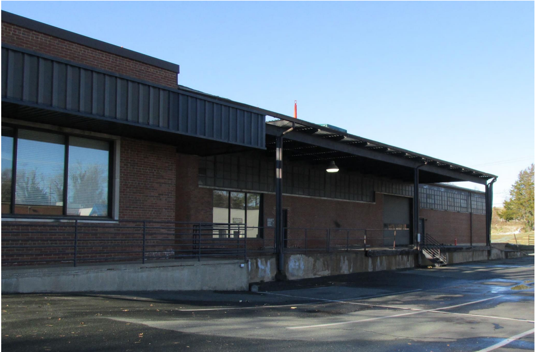
Figure 3: The east side of the building. The back portion that is to remain unchanged.
