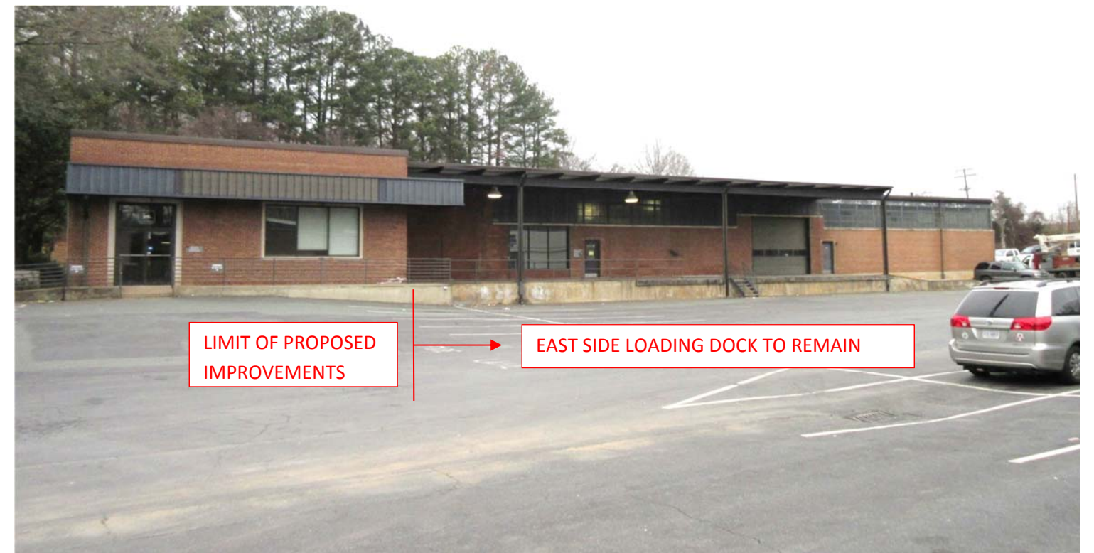
VIEW OF EAST SIDE ELEVATION
